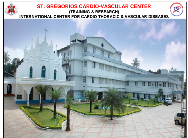
ST. GREGORIOS CARDIO-VASCULAR CENTER (TRAINING & RESEARCH) INTERNATIONAL CENTER FOR CARDIO THORACIC & VASCULAR DISEASES St. Gregorios Cardio-Vascular Center, Parumala Promoted by Frontier Lifeline, Chennai
